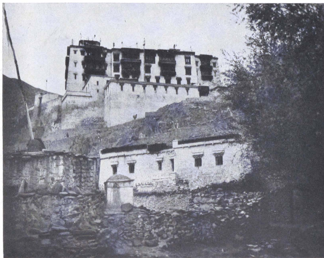
THE ROYAL SUMMER PALACE AT STOG, NEAR LEH—IT'S A WALK-UP CAN'T BE HEATED, NEEDS REPAIRS—BUT THE SCENERY IS MAGNIFICENT!
